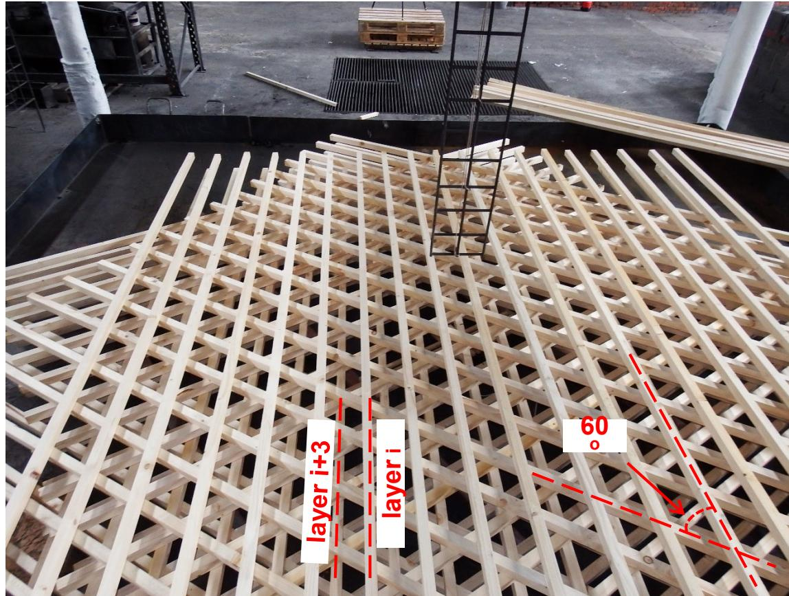
Figure 3. Wood stick arrangement in plan view: wood sticks orientation shifted  $60^\circ$  every layer, and every three layers wood sticks shifted horizontally for half of wood stick pitch.
